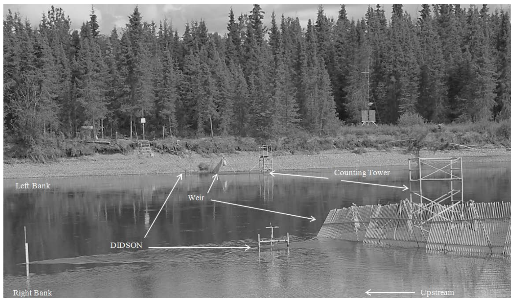
Figure 7.—Anvik River sonar project site (2016) illustrating locations of sonars, weirs, and counting towers.
